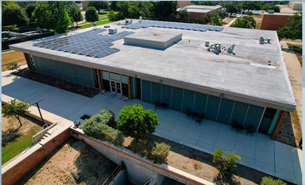
UIW School of Osteopathic Medicine Library rooftop solar installation. Source: https://www.uiw.edu/news/2025/09/uiw-school-of-osteopathic-medicine-commissions-rooftop-solar-project.html
